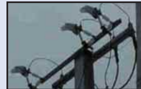
Overheated hinge on disconnect
