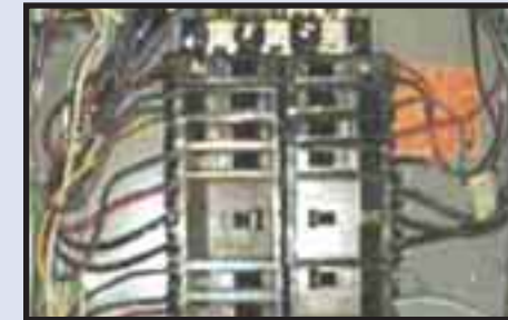
Poor connection and overloaded breaker
