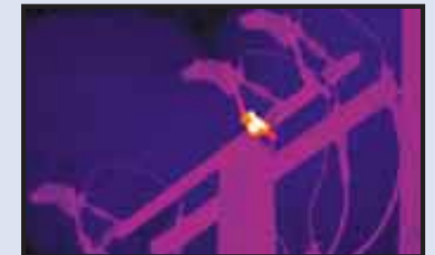
Overheated hinge on disconnect
